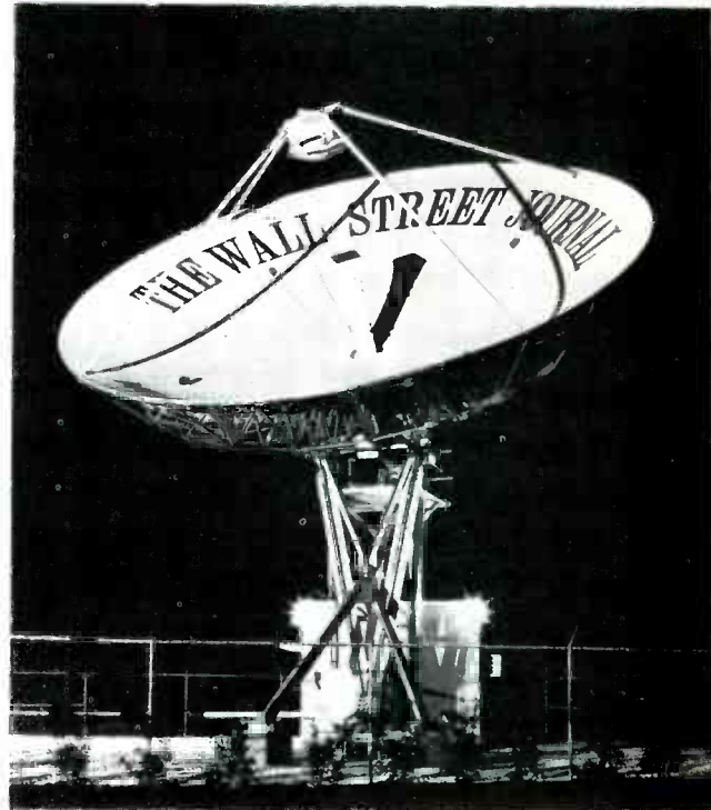
The Wall Street Journal newspaper operates this direct-reception terminal, so type set in Massachusetts can be printed in Florida. (Courtesy of American Satellite Corporation)
