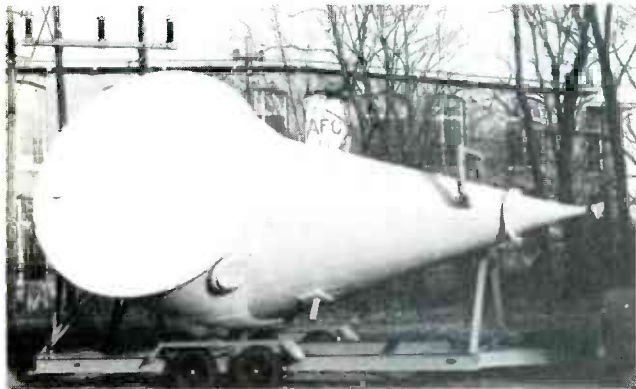
A 10' conical-horn antenna, mounted on a boat trailer, was used to receive MUSAK programs. Five other demonstrations also were successful, some operating from a 4' dish antenna. (Courtesy of Antennas For Communications, Inc.)
